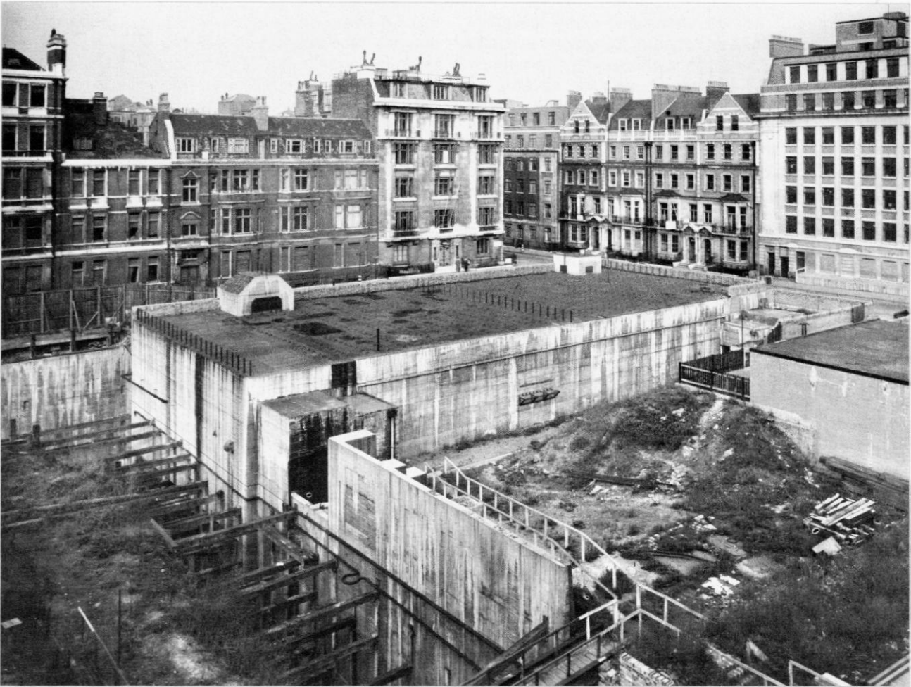
The Stronghold was a complete broadcasting centre in miniature built next to Broadcasting House during the war. In this view dated November 1945 the 9ft 6in-thick concrete roof (removed later to facilitate building the subsequent Broadcasting House extension) is clearly visible. The picture, looking north-east with Duchess Street on the left and Hallam Street on the right, shows protected air and exhaust vents, with a rectangular vent into the corridor. The protected porches have been removed but a temporary single-storey building is visible, along with the much deeper shored excavation for the basement of the abandoned pre-war extension scheme. It is just possible to make out the low-level door at the bottom of the staircase, facing into the excavation. [BBC]
